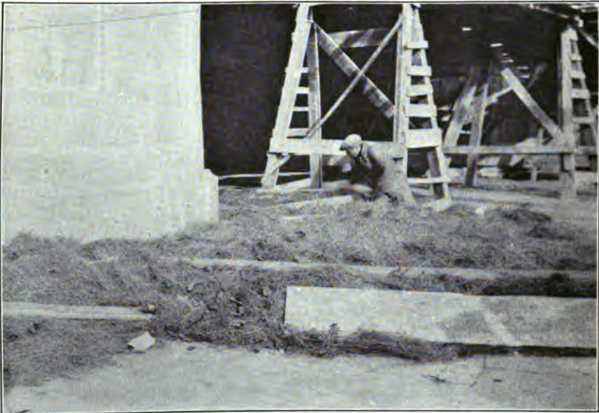
FIG. 7.—PROTECTING NEW-LAID SIDEWALKS AGAINST POSSIBLE DROP IN TEMPERATURE DURING THE NIGHT.
